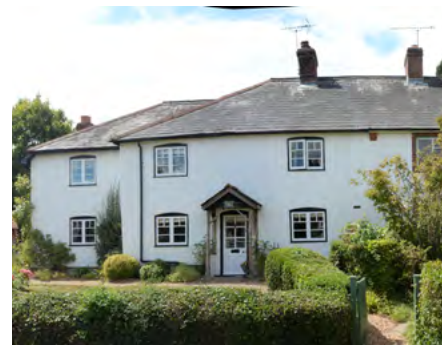
April Cottage extension.
